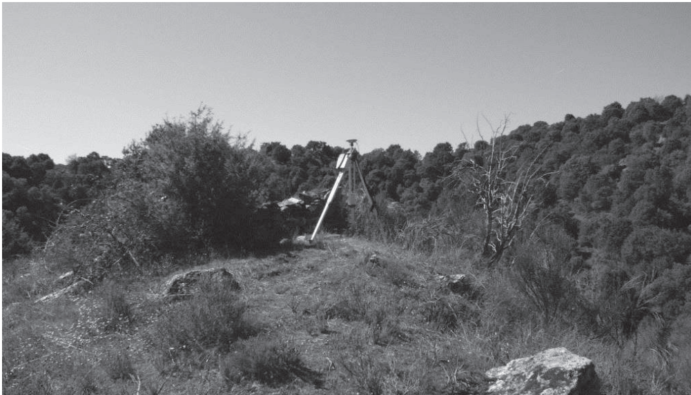
Figure 3 GPS receiver at the reference base near the dam
