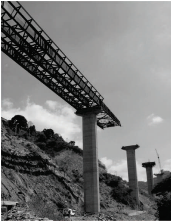
Figure 1 Incremental launching of the Viaduct Caracas-La Guaira (Venezuela)
