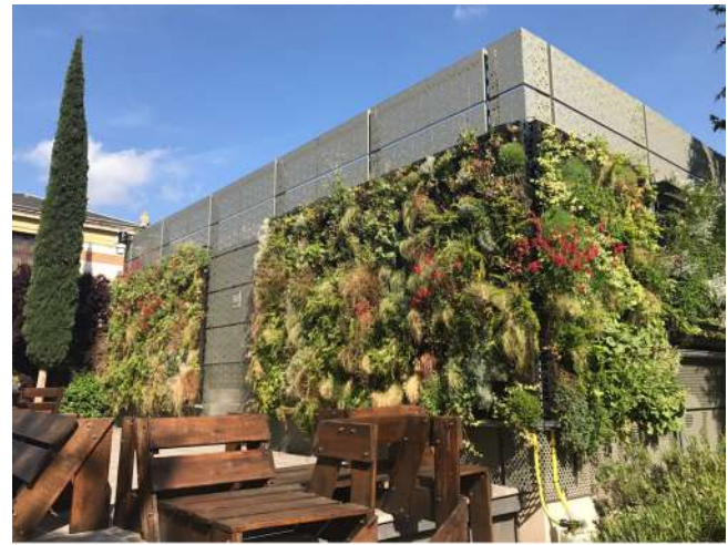
Figure 1 Headquarter of Innovation and Technology for Development Centre (itdUPM)
