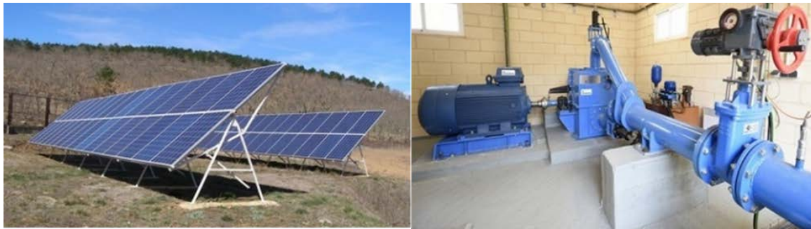
Figure 1 Photovoltaic turbine zone and Pelton turbine with 40 kW generator.
